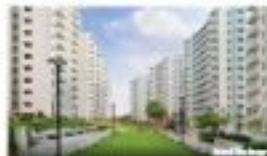
Godrej Gardens, Gurgaon
