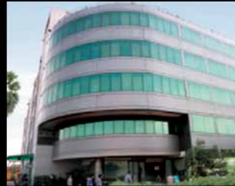
2003 BAANI - IBM, GURGAON
